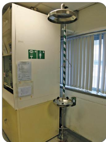
Figure 28: Safety shower with integrated eyewash and hand/ foot controls.
