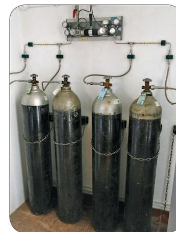
Figure 13: Gas cylinders secured in an upright position and stored in a cool, well-ventilated area.
